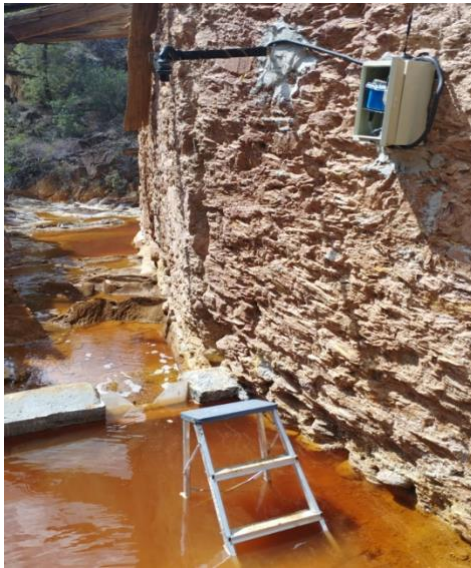
Water flow measuring station
