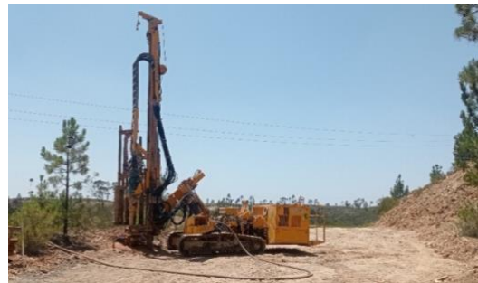
Equipment drilling the 40 m long hole for the piezometer
